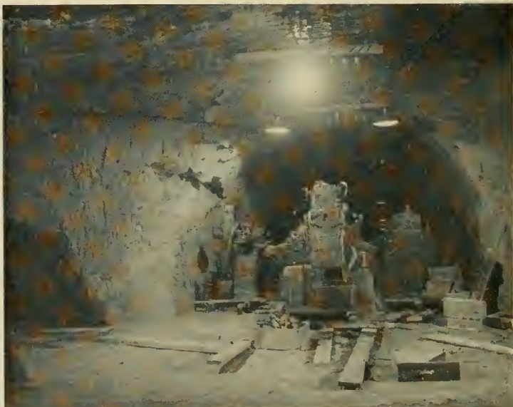
Photo No. 23.—Kukuri plant. Machine tools being installed.
