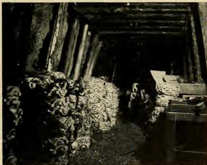
Photo No. 13.—Asakawa plant. Cross tunnel used for storage of engine parts.
