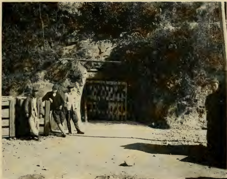
Photo No. 20.—Small tunnel used for installation of machine tools, Kukuri plant.
