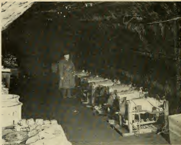
Photo No. 14.—Yokosuka plant, assembly tunnel.
