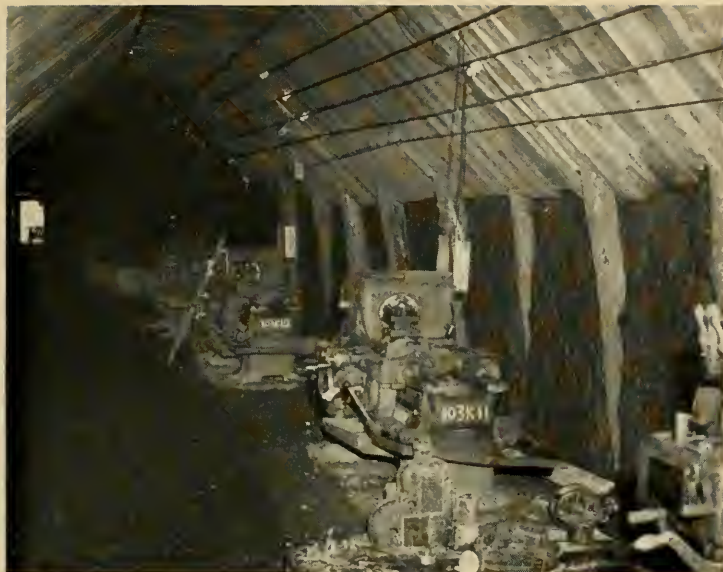
Photo No. 12.—Oami plant. Note lumber roof.
