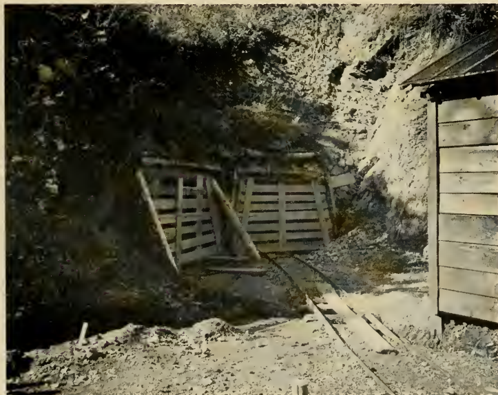
Photo No. 21.—Tunnels used for installation of machine tools, Asakawa plant. Note narrow gage track.
