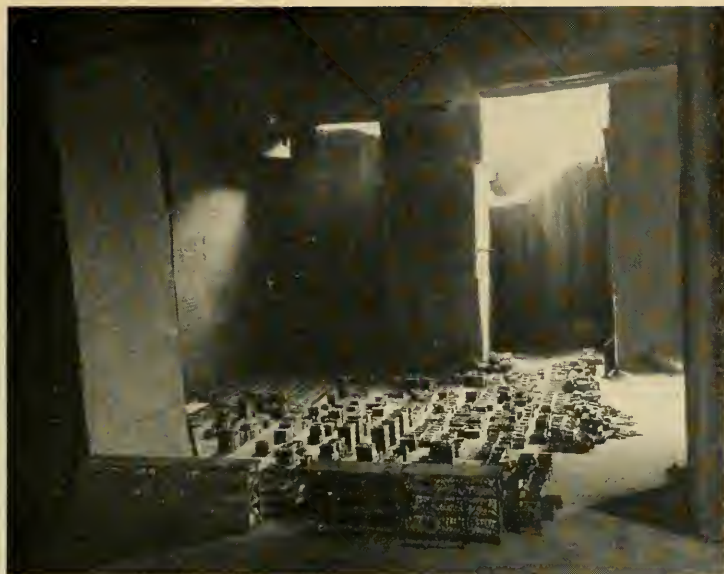
Photo No. 9.—Shiroyama plant, storage area.
