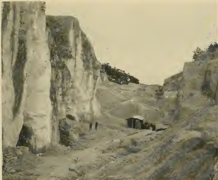
Photo No. 17.—Entrances to Yoshimatsu plant.
