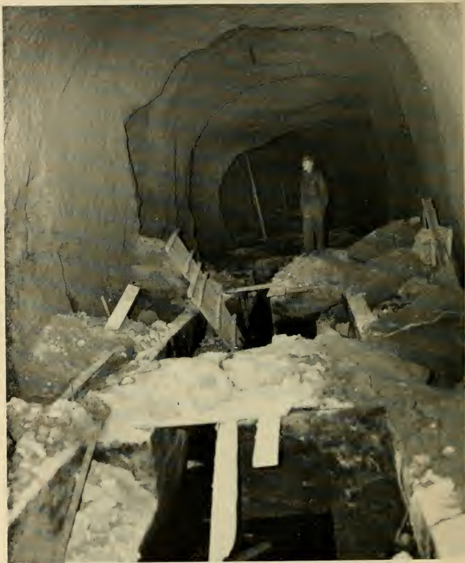
Photo No. 11.—Yoshimatsu plant, heat treatment pits under construction in foreground.
