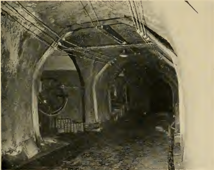
Photo No. 29.—Handa plant. Note production tunnels opening into communications tunnel.
