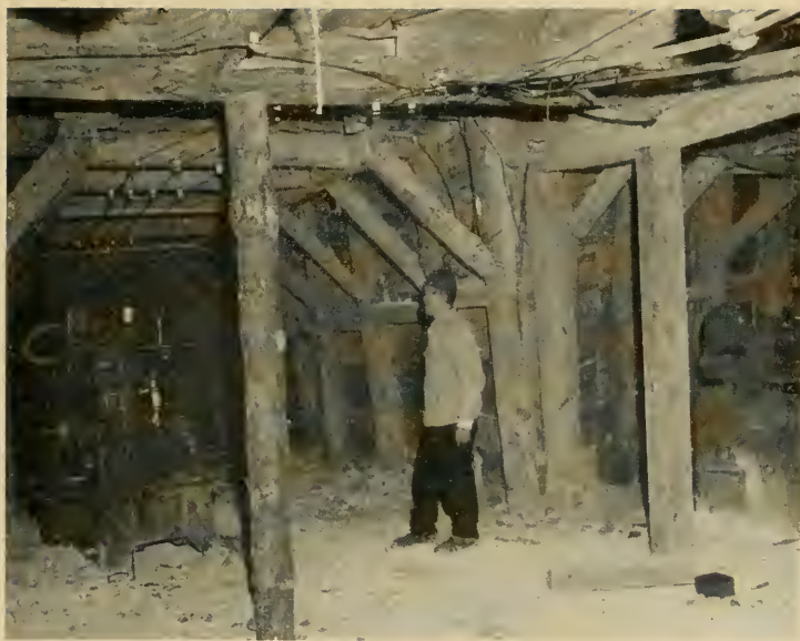
Photo No. 24.—Sero plant. Note extensive shoring.
